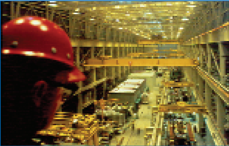
Most factory floors in North America are lit with industrial discharge lamps, such as sodium vapour or mercury vapour.
